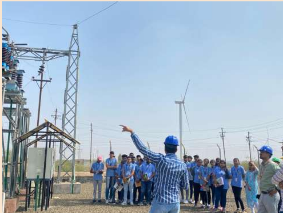
Renew Extra High Voltage Power Substation, Walsang road, Jath Sangali
