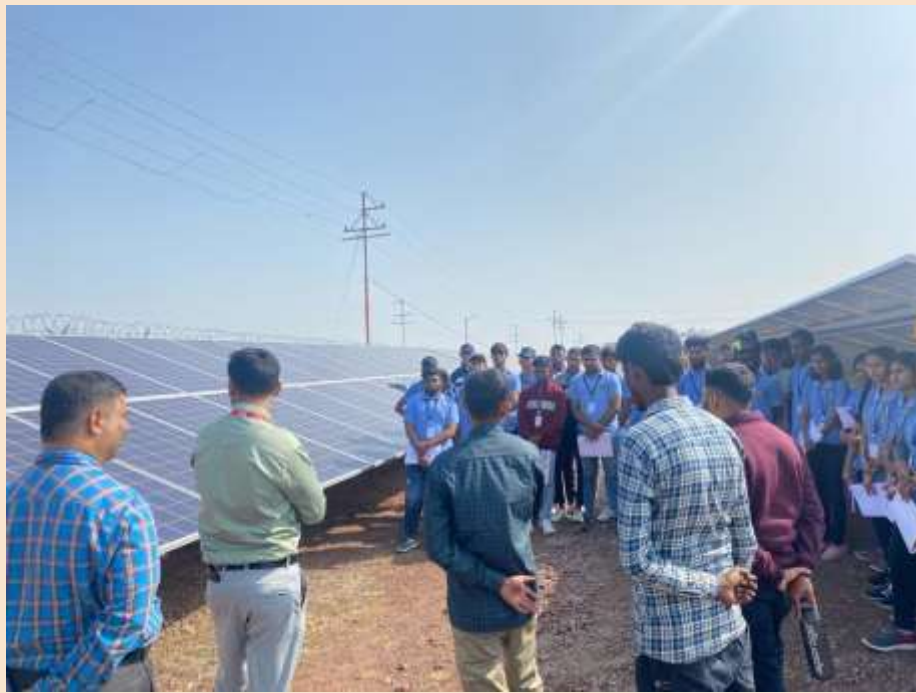
TATA solar power plant, Walekhindi, Jath Sangali1
